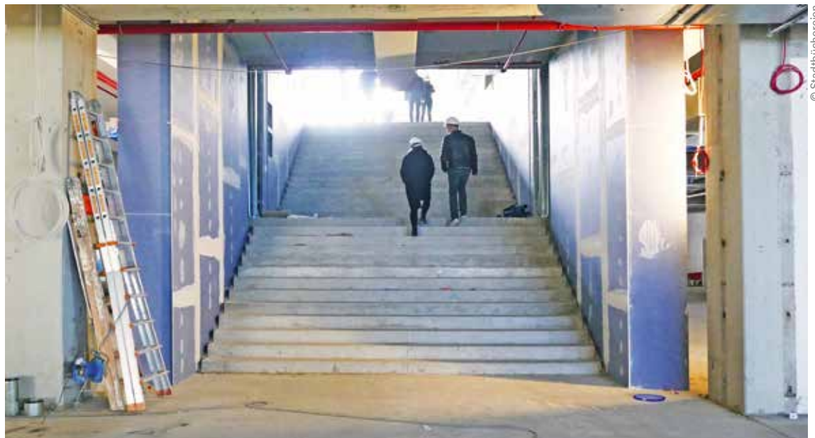
The entrance to the staircase under construction in 2020
